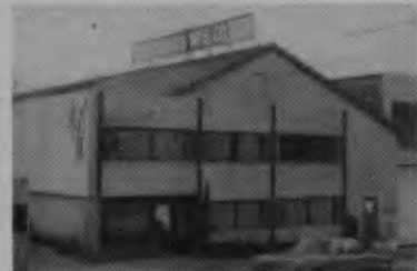
The Arcweld Manufacturing Company Factory will soon be the SPC Science Center.
