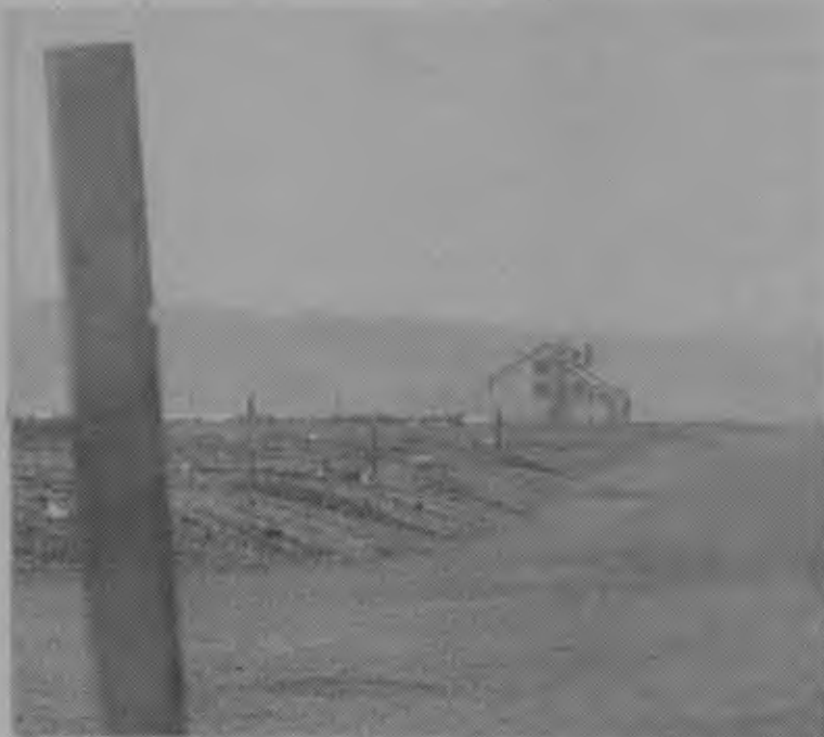
Two duplexes, graded roadways and imported gravel mark the area where dozens of structures are planned.
