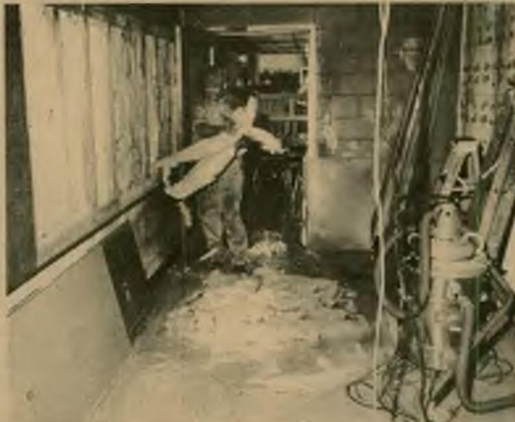
Peder Grambl, an employee of a local clean-up service, strips insulation from the walls of the Weter Library typing room where fire broke out Sunday.
